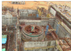
Kalpakkam FBR construction
